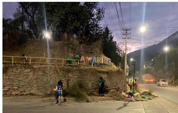
Av. Regional – Puente Huallaga
